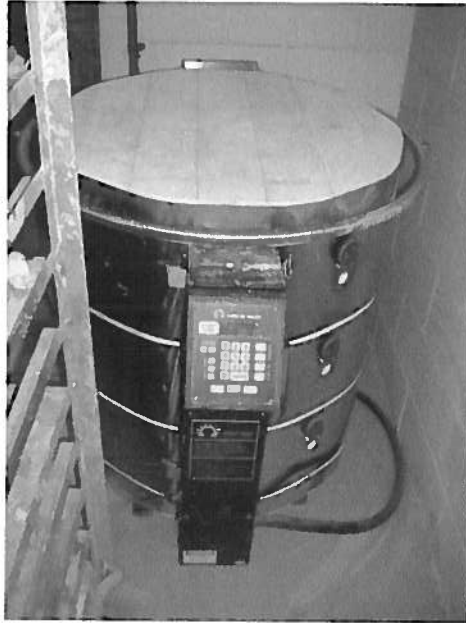
Photo 2: Suspected ACMs in the refractory linings of the two (2) kilns located in the kiln room (Room 18) at the Dovercourt Recreation Complex. (August 21, 2009).
