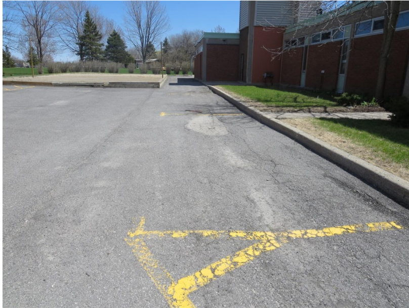
Photo 23: Driveway at north side
