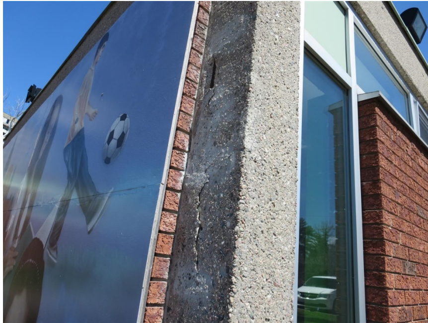
Photo 3: Concrete deterioration
