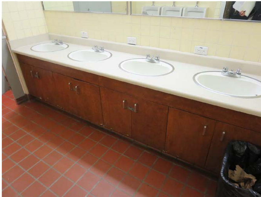
Photo 10: Finishes in Men's washroom
