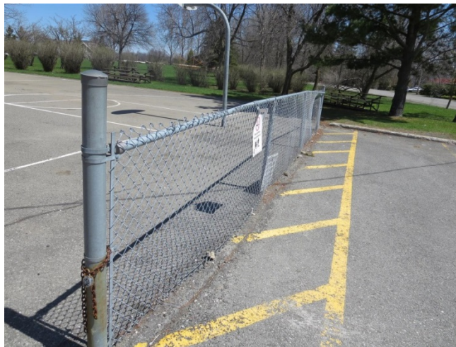
Photo 21: Chain link fencing.
