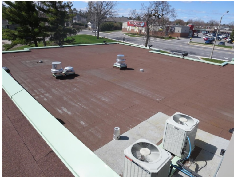
Photo 6: Lower roof – main building
