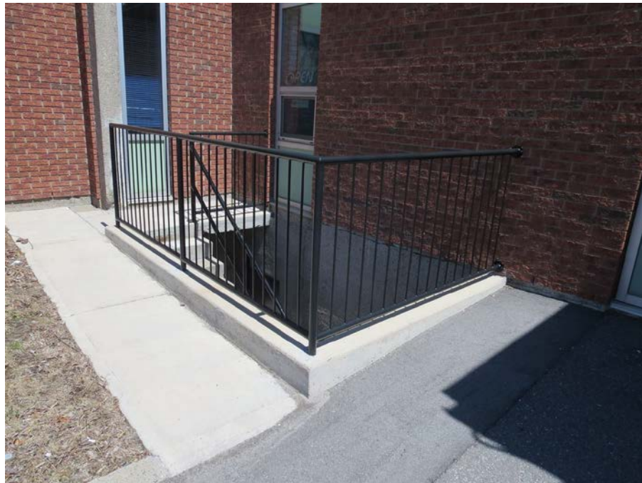
Photo 24: Concrete stairs to basement
