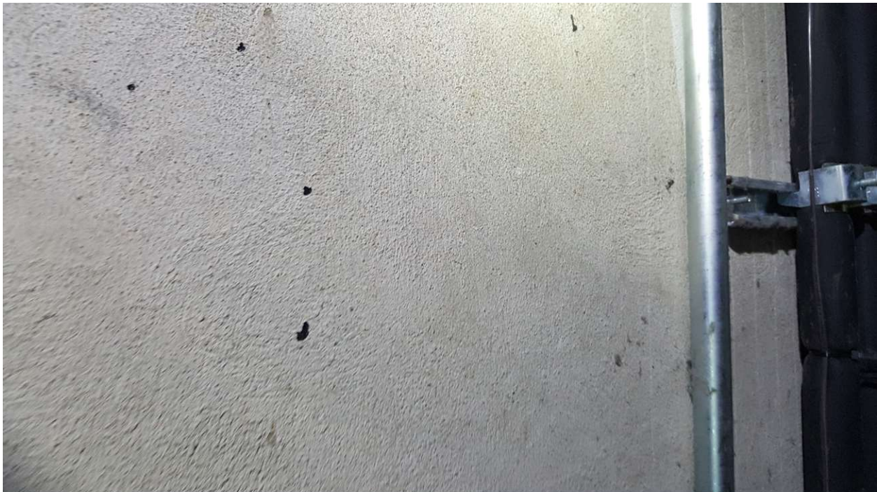
Photograph 5: Non-friable rough textured plaster, which contains 0.5% Chrysotile asbestos, observed on the walls of the former bell tower.
