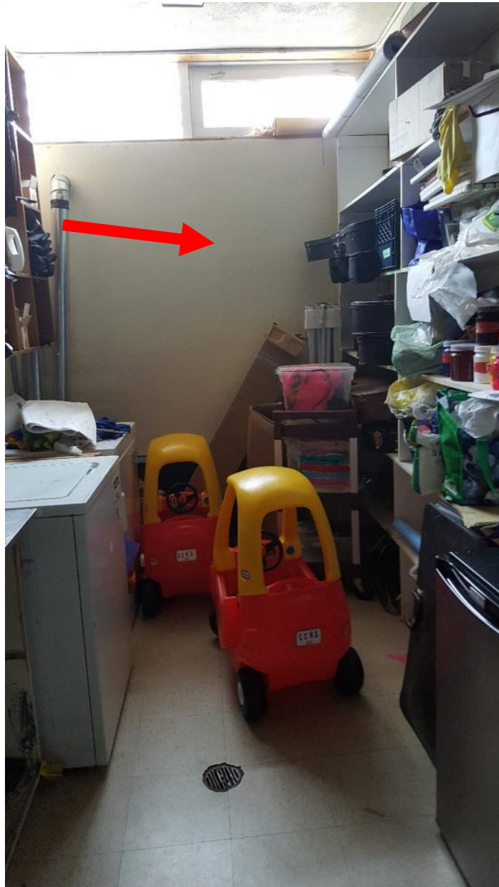
Photograph 6: Non-friable rough textured plaster, which contains 0.5% Chrysotile asbestos, observed on the walls of the rooms north of the gymnasium.
