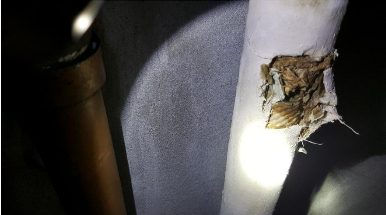
Photograph 9: Friable cardboard wrap pipe straight run insulation which contains 5% Chrysotile asbestos (DST Sample 12A-C) were observed in the basement south-east and south/middle storage rooms.
