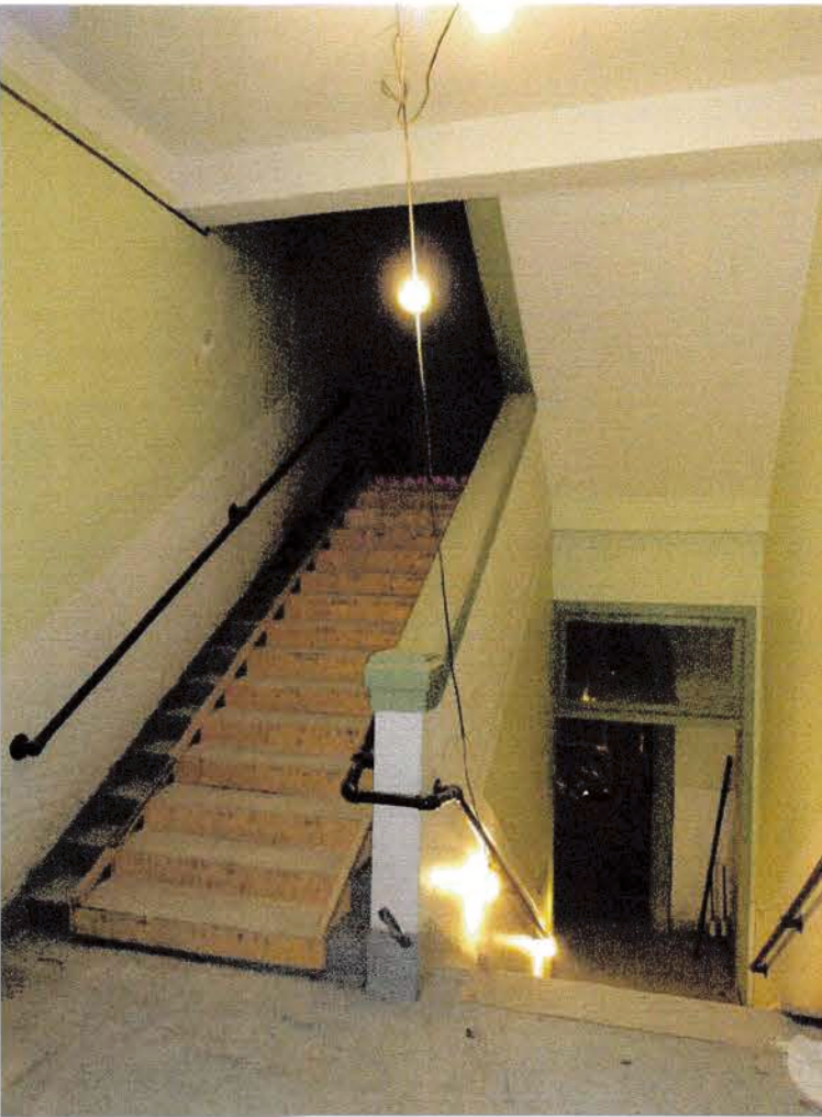
1 STAIRWELL WOOD TRIM
