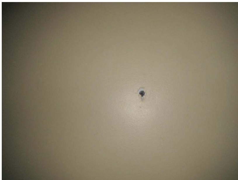
Photo 29: View of Representative Asbestos Containing Plaster, Main Building, Ground Floor Corridor, Sample Set: PL-3-X.
