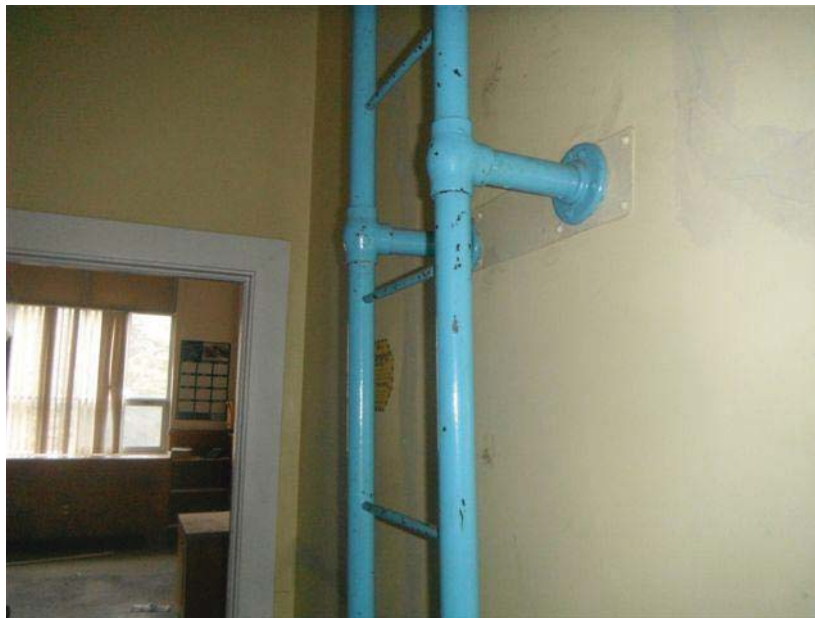
Photo 51: View of Representative Lead Containing Blue Ladder Paint, Main Building, Room 014, Sample: LBP-I.
