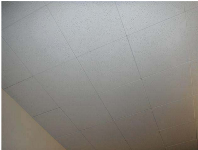
Photo 39: View of Representative Asbestos Containing 1'x 1' Ceiling Tile, Main Building, Room 006, Sample Set: CT-6-X.
