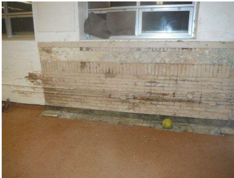
Photo 55: View of Moisture Impacted Wall, Evidence of Moisture Infiltration, Main Building, Library.
