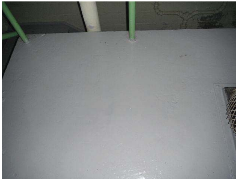
Photo 45: View of Representative Lead Containing Grey Floor Paint, Annex Building, Mechanical Room, Sample: LBP-C.
