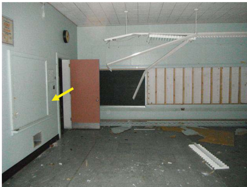
Photo 46: View of Representative Lead Containing White Wall Paint, Annex Building, Room 004, Sample: LBP-D.
