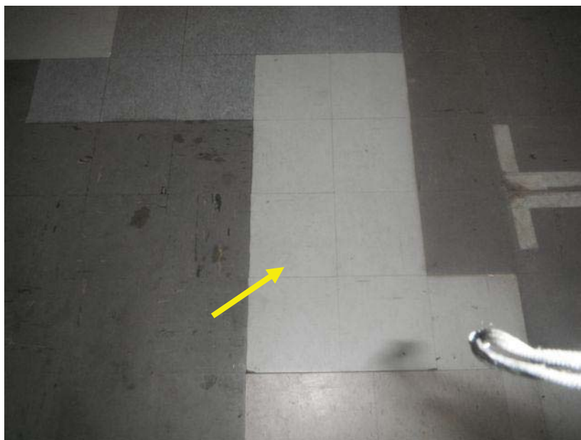
Photo 36: View of Representative 9" x 9" White Vinyl Floor Tile with Asbestos Containing Mastic, Main Building, Room 007, Sample Set: VT-11-X.
