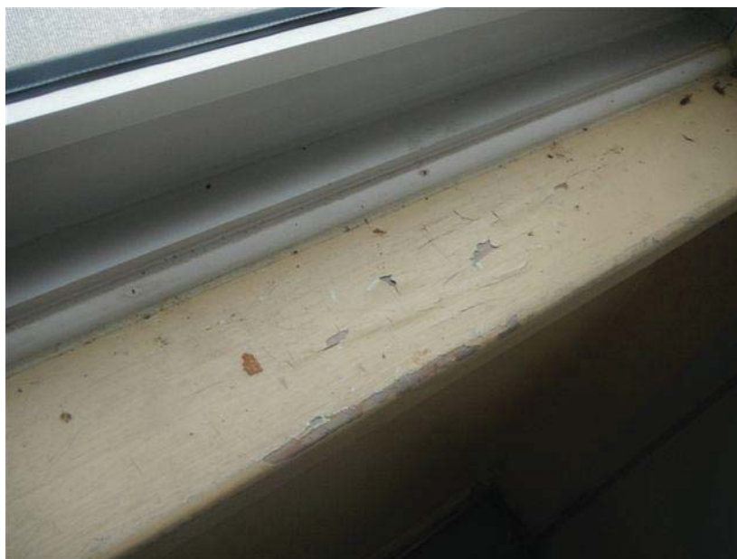
Photo 50: View of Representative Lead Containing Yellow Window Frame Paint, Main Building, Room 006, Sample: LBP-H.
