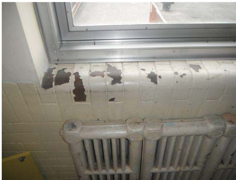
Photo 52: View of Representative Lead Containing Yellow Wall Paint, Main Building, Room 004, Sample: LBP-J.
