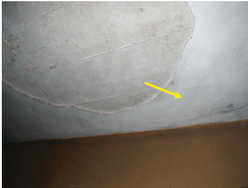
Photo 27: View of Representative Asbestos Containing Plaster located on Concrete, Main Building, Storage Room, Sample Set: PL-2-X.
