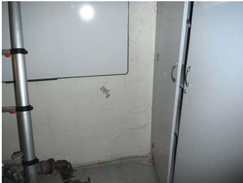
Photo 47: View of Representative Lead Containing Beige Wall Paint, Main Building, Kitchen, Sample: LBP-E.
