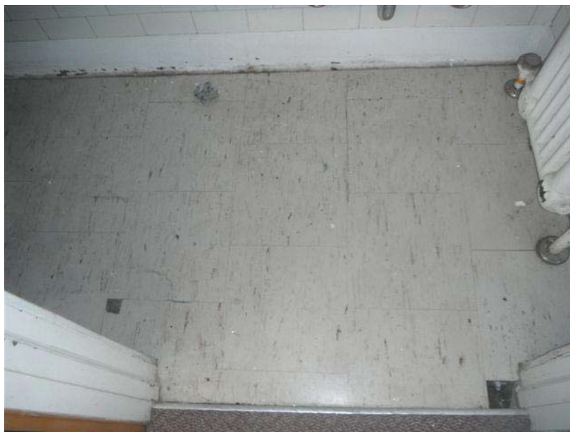
Photo 40: View of Representative Asbestos Containing 1'x 1' Beige Vinyl Floor Tile, Main Building, Room 006, Sample Set: VT-12-X.
