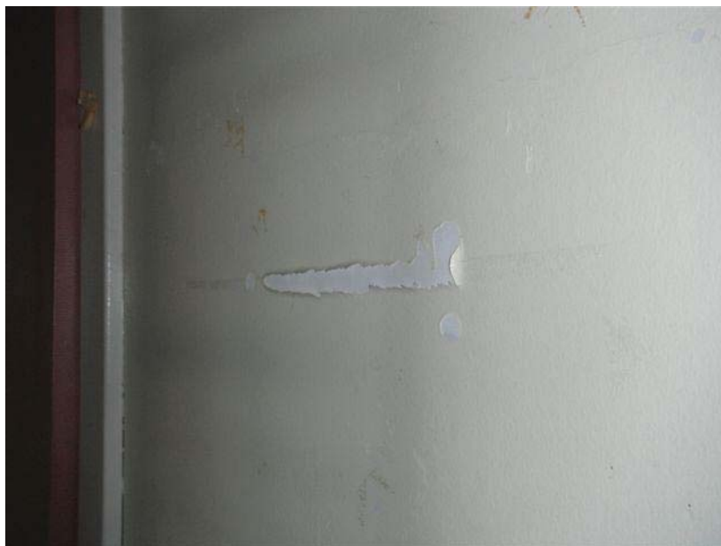
Photo 43: View of Representative Lead Containing Beige Wall Paint, Annex Building, Room 004A, Sample: LBP-A.
