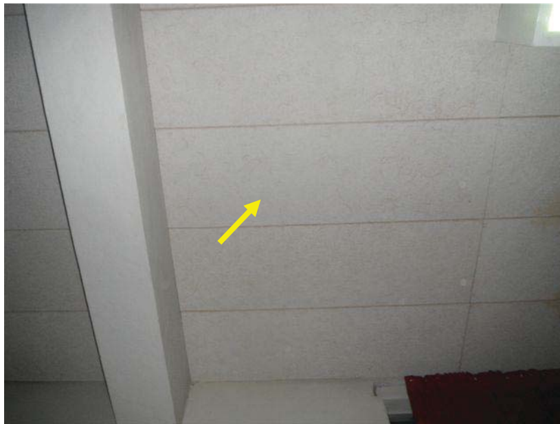
Photo 53: View of Representative Potential Asbestos Containing Ceiling Mesh-like Panels, Main Building, Gymnasium. Inaccessible during initial assessment.
