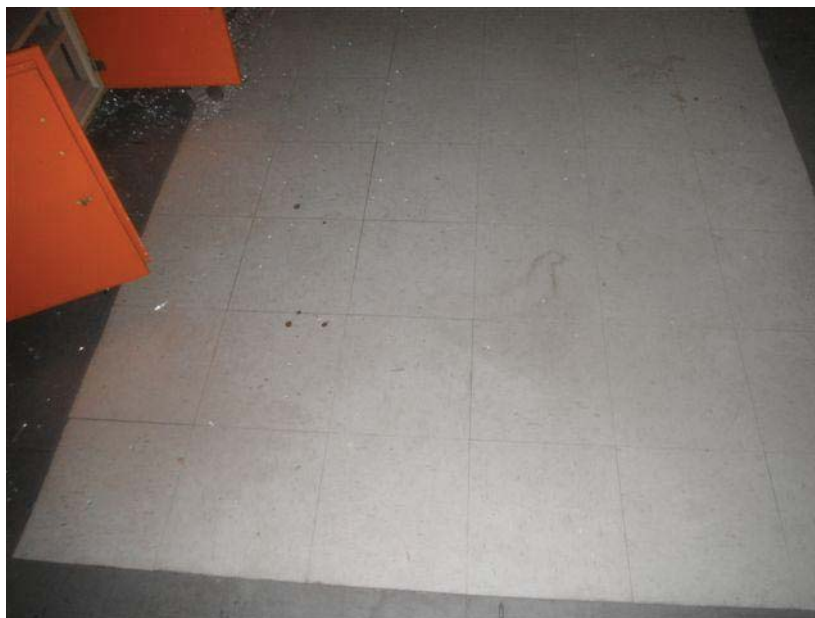
Photo 35: View of Representative 1' X 1' White Patterned Vinyl Floor Tile with Asbestos Containing Mastic, Main Building, Room 007, Sample Set: VT-10-X.
