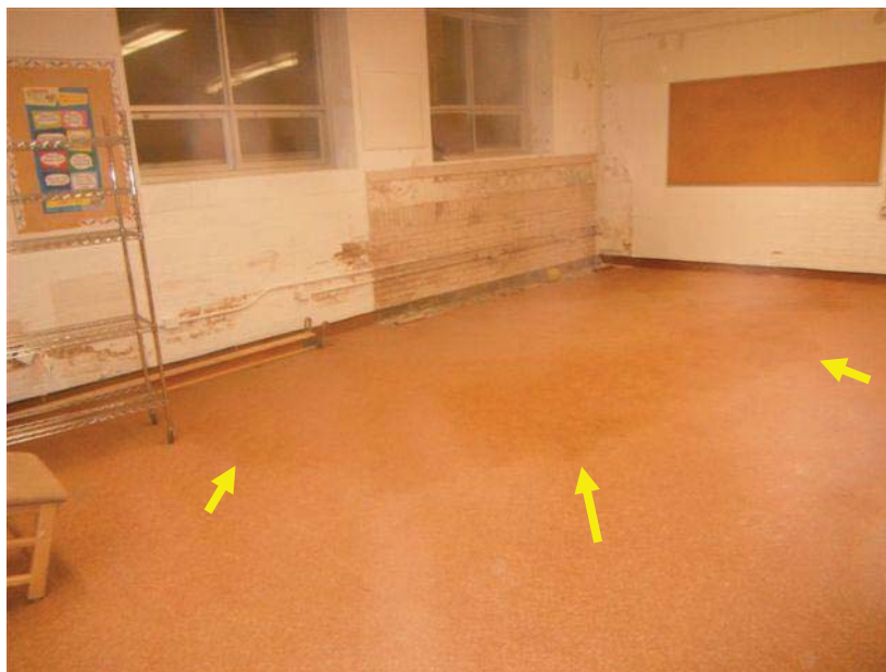
Photo 54: View of Moisture Impacted Carpet, Evidence of Moisture Infiltration, Main Building, Library.
