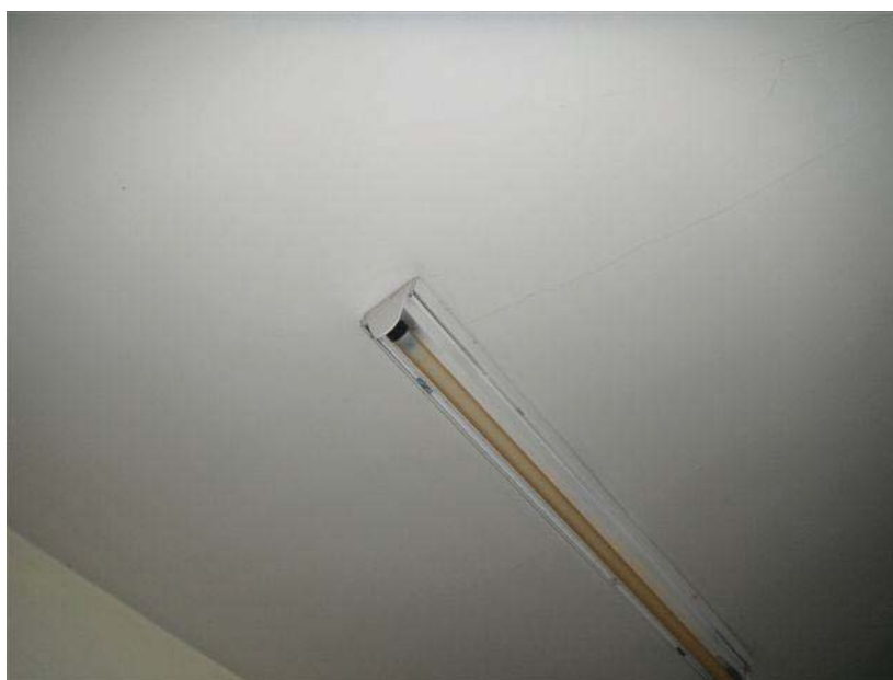
Photo 44: View of Representative Lead Containing White Ceiling Paint, Annex Building, Waiting Room, Sample: LBP-B.
