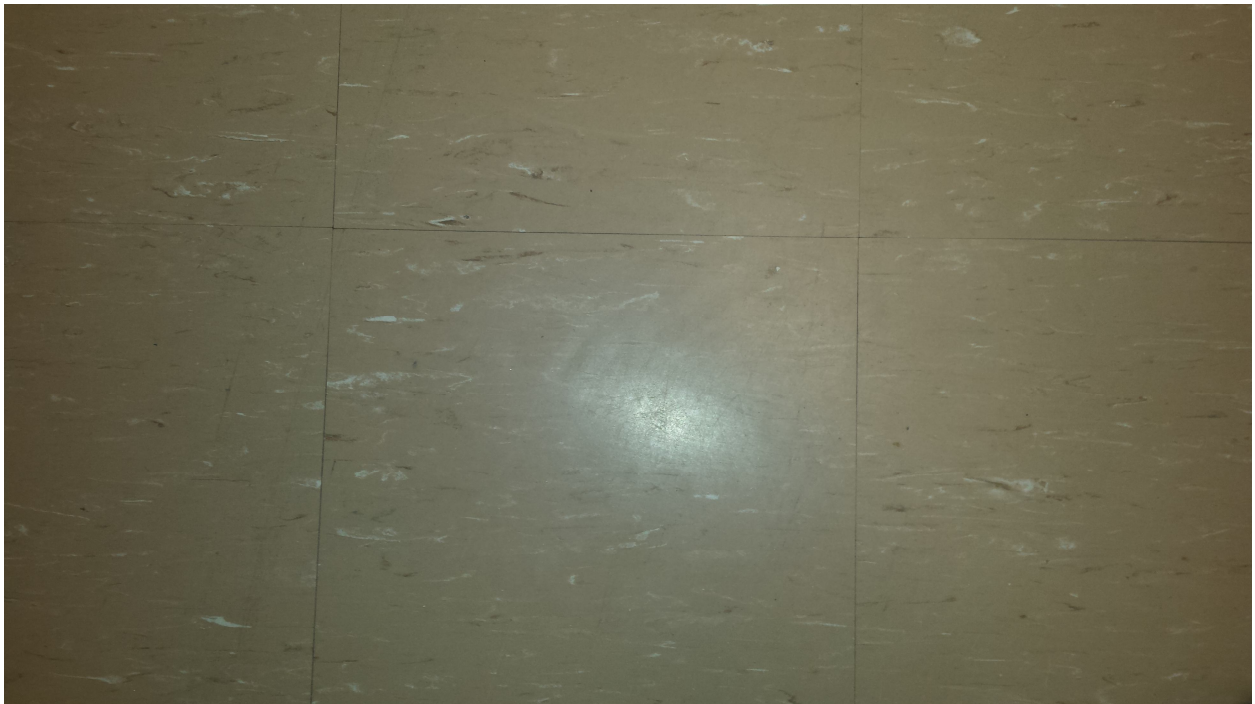
Photo 4 – View of asbestos 30cm x 30cm vinyl floor tile.
