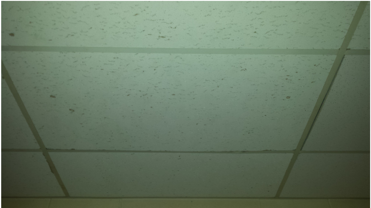
Photo 3 – View of asbestos 60cm x 120cm ACM ceiling tiles.
