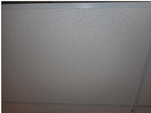
Non-asbestos ceiling tiles present throughout the assessed area.
