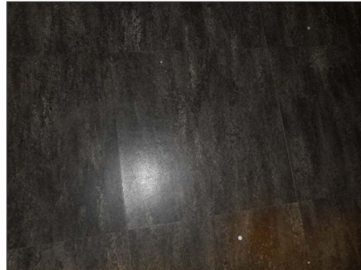
Non-asbestos 12" black vinyl floor tiles with a stone pattern.
