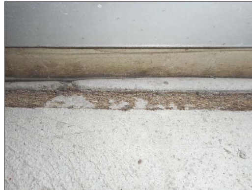
Non-asbestos grey exterior caulking.
