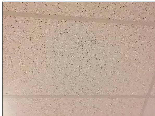
Non-asbestos, 2'x4' lay-in, random pinhole acoustic ceiling tile.
