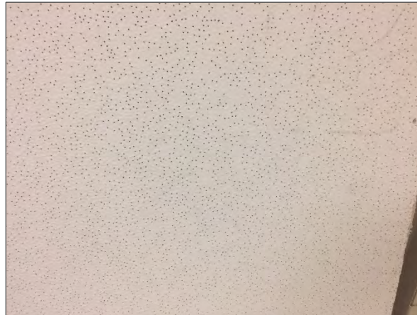
Non-asbestos, 2'x4' lay-in, small pinhole acoustic ceiling tile.
