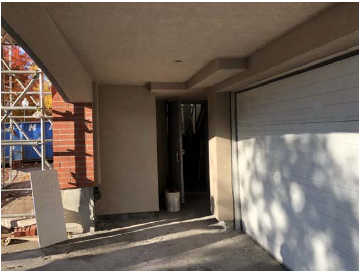
07 Soffit at Garage Entry
