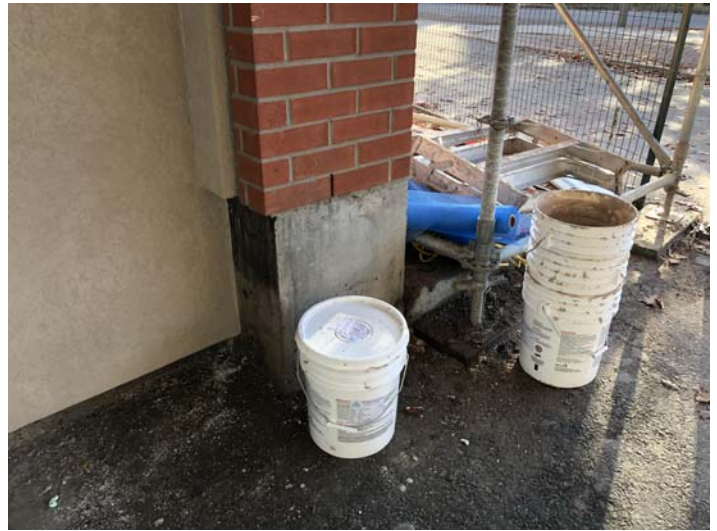
14 Damaged Parging at South Pier
