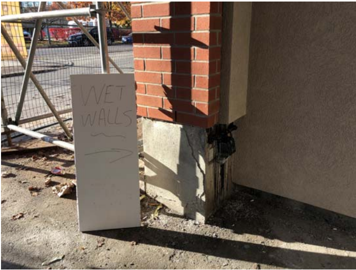
13 Damaged Parging at North Pier
