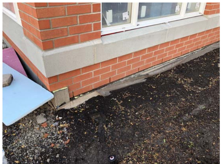
06 Base of North Wall
