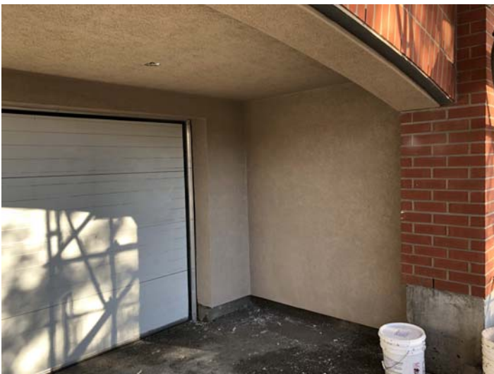
11 EIFS at Garage Entry
