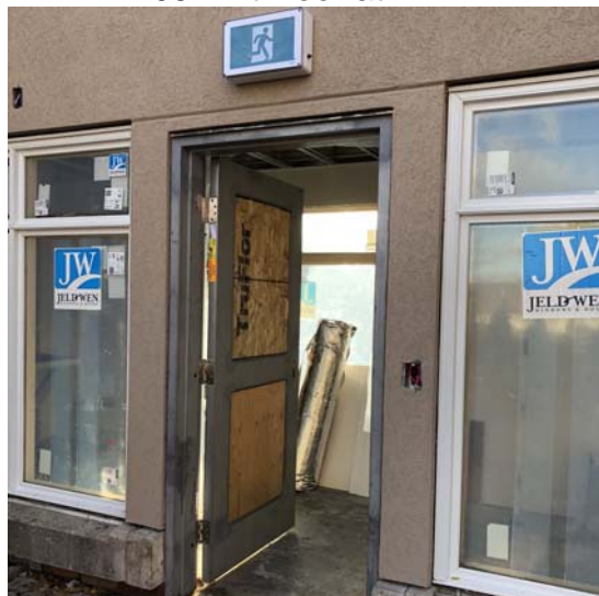
05 Exit Door at Link
