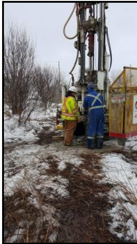
Photograph 1: View of the advancement of borehole BHMW16-6, facing southeast (March 8, 2016)
