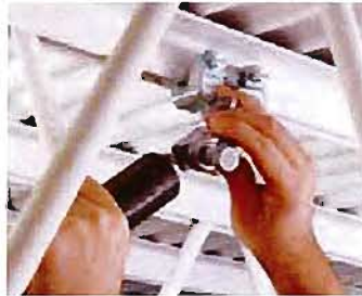
Step 1: Mount Universal Structural Attachment to chosen structural attachment (concrete, Bar Joist Adaptor, I-Beam Adaptor or other structural element).
