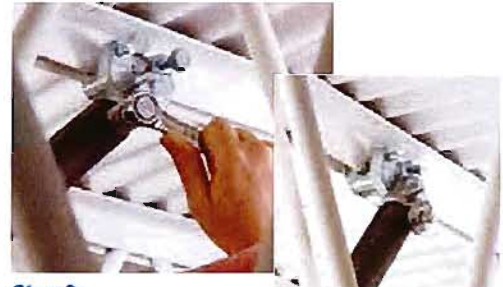
Step 2: Insert brace pipe and tighten shear bolt until head snaps off.
