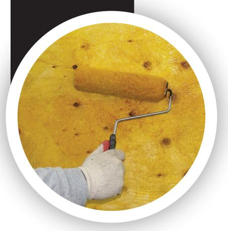
**IKO S.A.M. Adhesive** should always be used in well-ventilated conditions and kept away from all sources of potential ignition.
