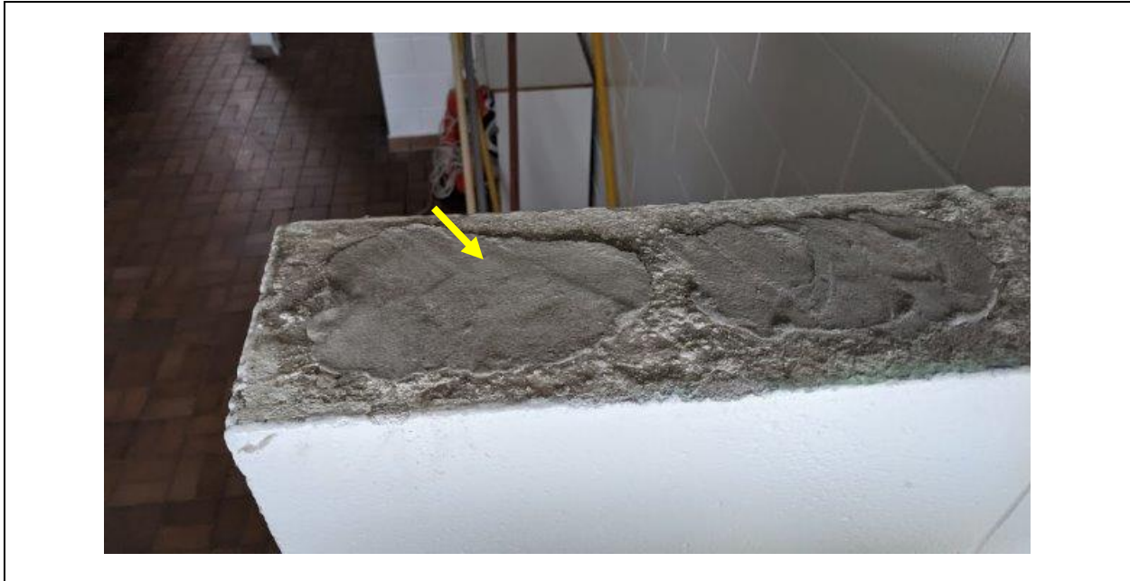
Picture 3: Concrete Block Filler, Interior Concrete Blocks, Sample Set: CF-1
