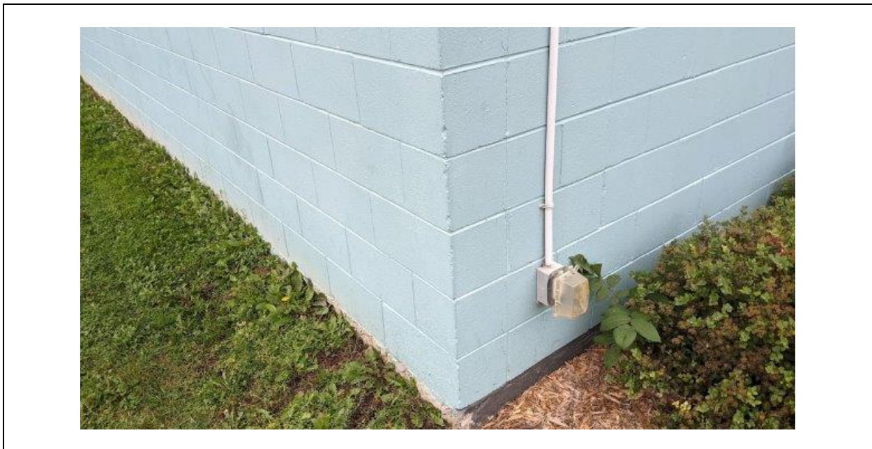
Picture 6: Paint, Aqua Blue, Throughout Site, Sample: LP-1
