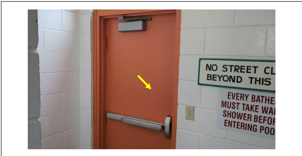
Picture 8: Paint, Orange, Doors, Framing, Sample Set: LP-3
