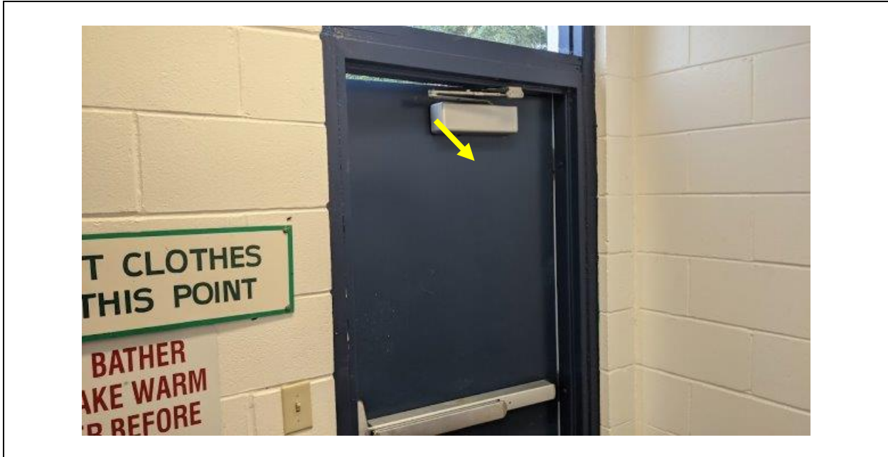
Picture 9: Paint, Dark Blue, Doors, Framing, Sample: LP-4
