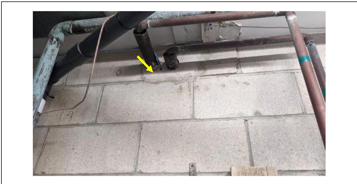
Picture 4: Parging, Utility Penetrations, Sample Set: PA-1
