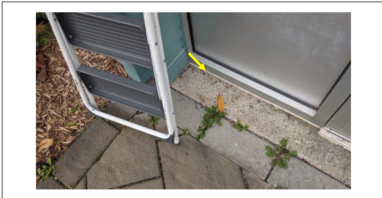
Picture 1: Caulking, White Colour, Site Exterior, Sample Set: CK-1
