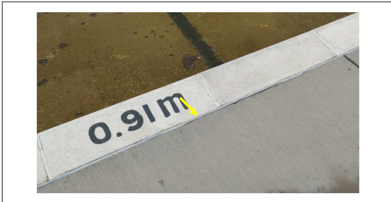
Picture 2: Caulking, Grey Colour, Site Exterior, Sample Set: CK-2
